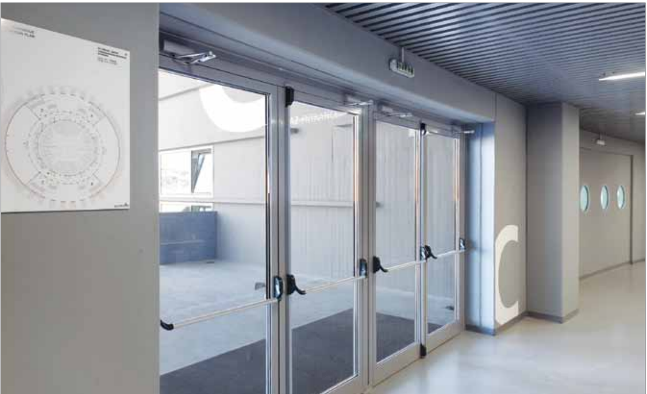
Sports hall, Zadar, Croatia (Photo: Robert Les)
